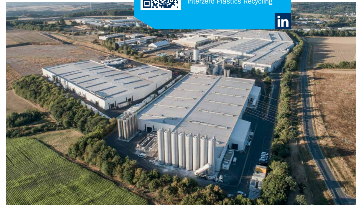
CLASSEN Group production plant in Kaisersesch: where the sustainable material CERAMIN® is made
